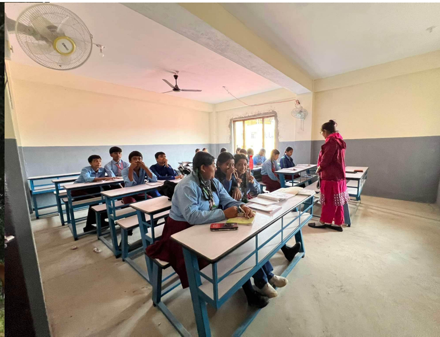
Classroom repair and maintenance
